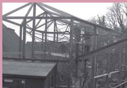
Work on the 'Back' enclosure continued in all weathers.
